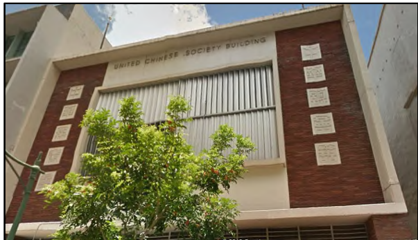
UCS Building at 42 N. King Street
